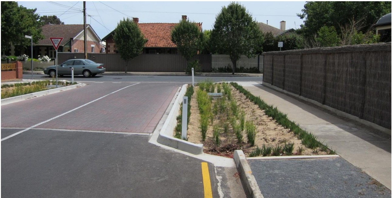
Figure 14 Typical Bioretention garden soon after planting
