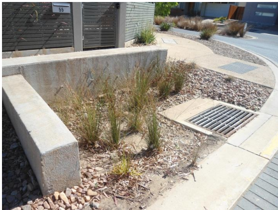
Figure 1: Bioretention basin in Lochiel Park
