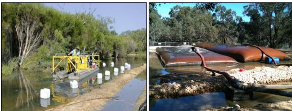
Figure 13. Micro-dredge in operation (left) and desludging tubes (right) (from Simpson et al. 2018 – case study in national guidance for dredging of acid sulfate soils document).
