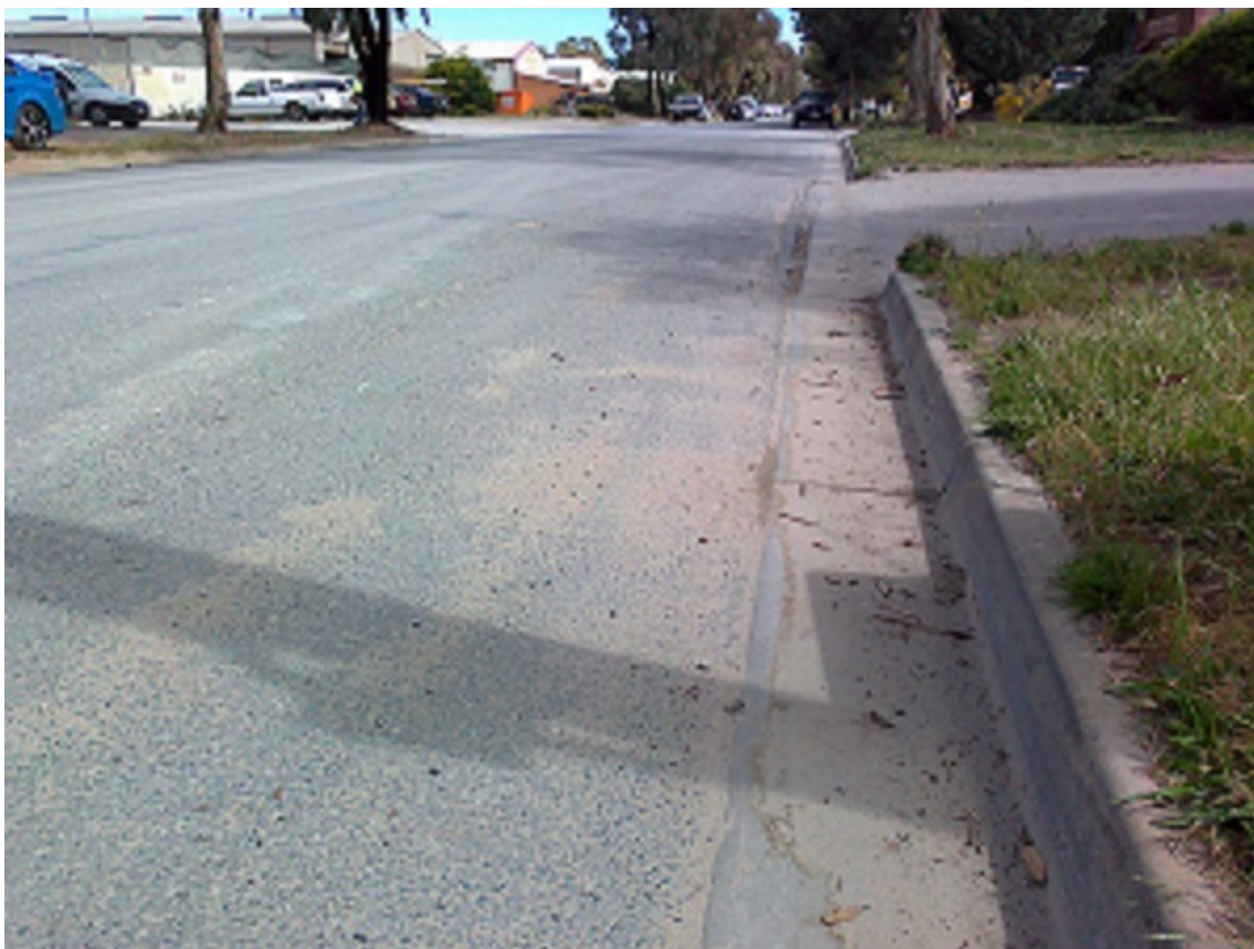
Figure 10 Road with sand, cement and other debris in the Parafield catchment next to a cement factory.
