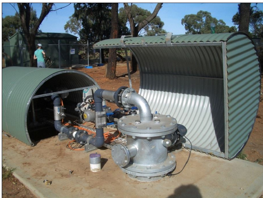
Figure 12 Production well at Parafield ASTR site showing injection and extraction pipework, flow meter (totaliser) and lockable enclosure.
