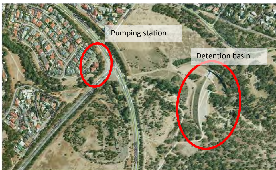
Figure 2-2 – Aerial photograph of the Cobbler Creek retention basin, indicating where flows are pumped into the Parafield catchment on the left and the temporary detention basin on the right (image courtesy of Googlemaps, 2010)
