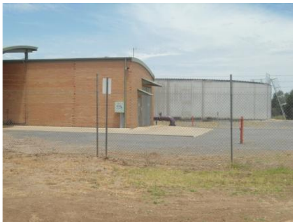
Figure J-17- (a) Recycled water mixing station at Greenfields for Mawson Lakes supply (b) the recycled water is used for toilet flushing , gardens and public open space irrigation
