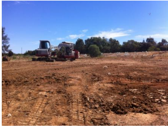
Figure J-19- (a) Greenfields wetland during summer (b) sediments cleared off from a sedimentation basin
