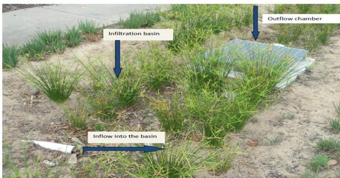
Figure J-40- Components of a typical raingarden in Mile End
