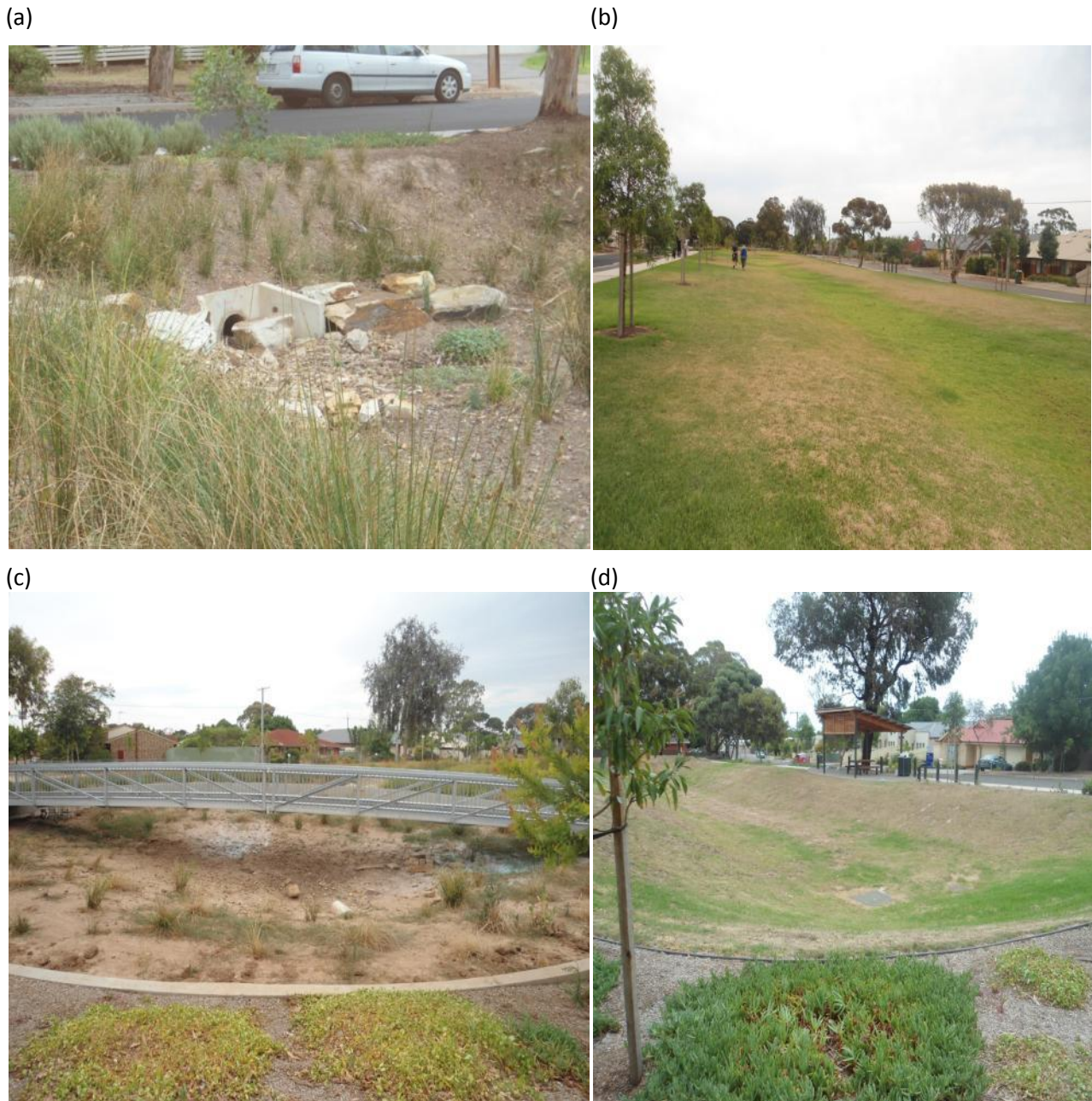
Figure J-14- WSUD features in the reserve (a) inlet (b ) turf basin (c) pond (d) detention basin
