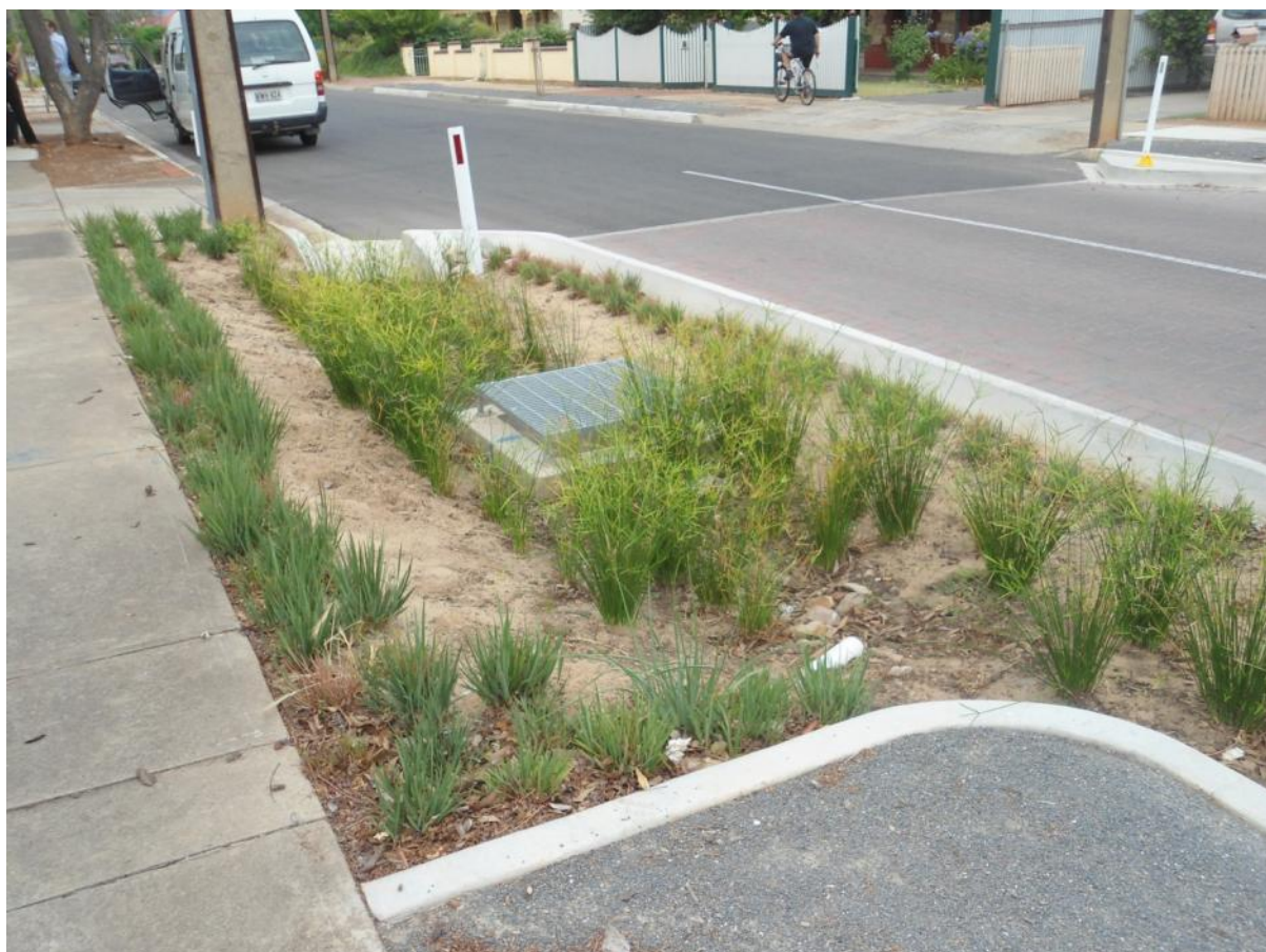
Figure 8-4- Rain-garden system at Mile End
