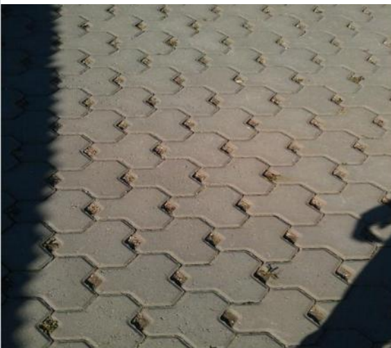
(e) Permeable Paver at on back street, City of Unley
