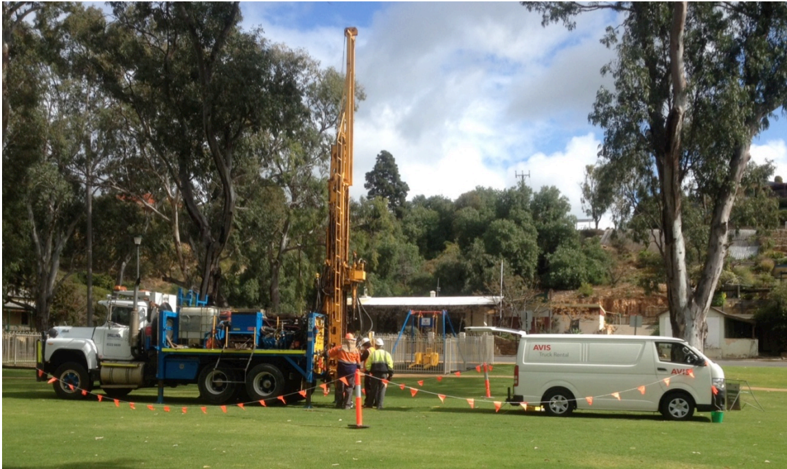
Figure 38: CPTu testing was undertaken at Mannum.
