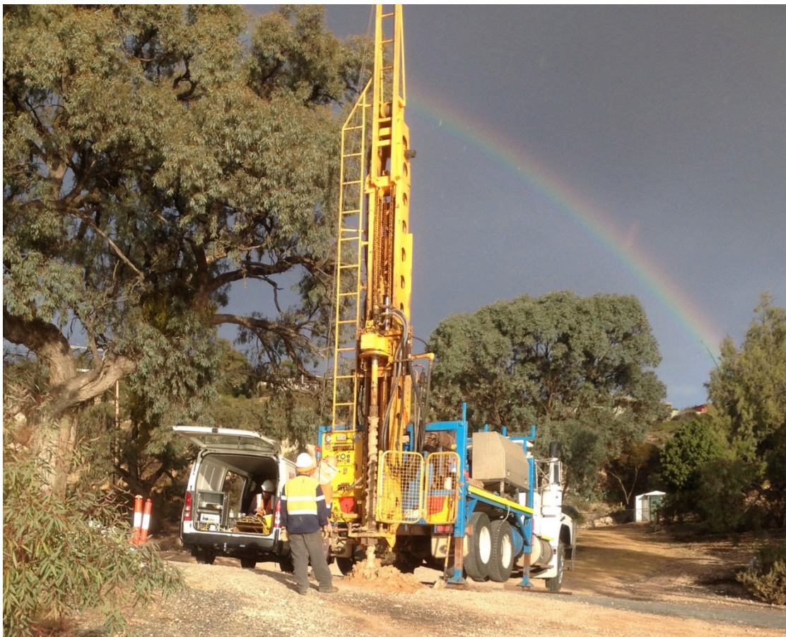
Figure 39: Relief drilling for CPTu testing at Nildottie.
