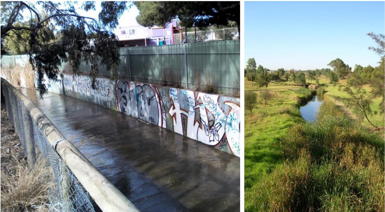
Figure 2. A typical example of an open concrete drain (Morphett Vale, SA) compared to a natural channel arrangement (Mawson Lakes, SA).
