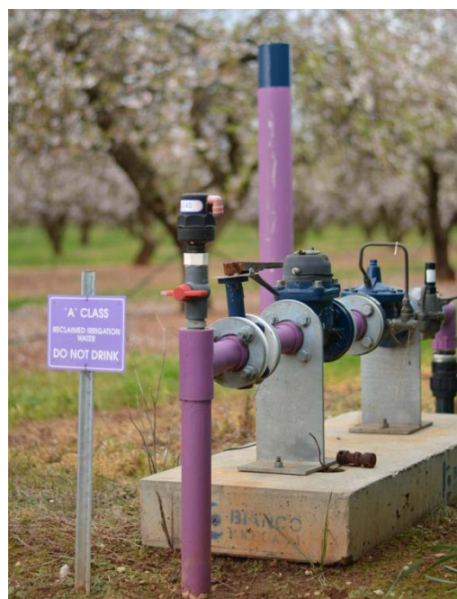
Figure 20. Recycled wastewater irrigation headworks at NAP almond orchard.
