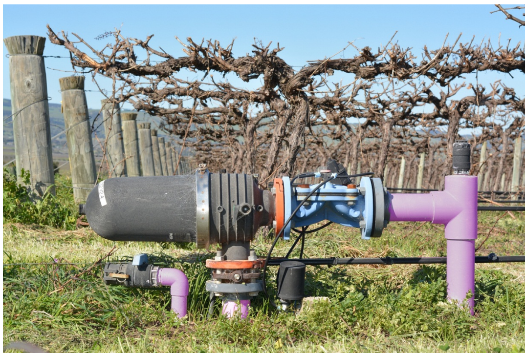
Figure 2. Recycled wastewater irrigation headworks at McLaren Vale Cabernet Sauvignon trial site.
