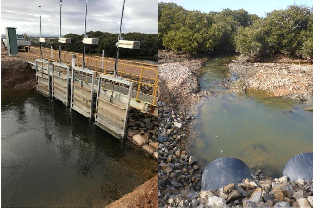
Figure 5. Tidal gate infrastructure showing the controllable gates (left) and the polyethylene pipes connecting the trial pond to pumping creek and mangroves in Barker Inlet (right). Photos Luke Mosley and Sabine Dittmann.
